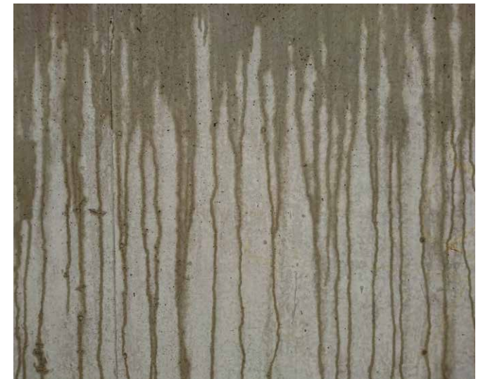
Traditional silanes on vertical surfaces are prone to excessive run-off. Excessive run-off leads to low penetration, significant material loss and poor performance.
